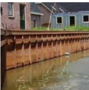
houten beschoeiing
